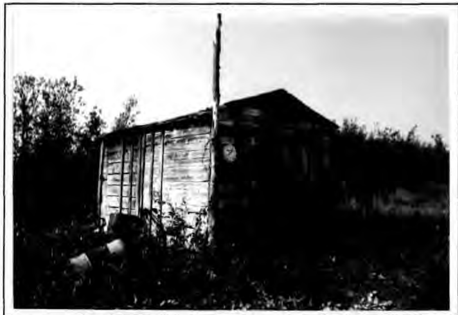
Figure 102. The Airstrip Storage Shed, 1993. The view is looking southwest.
